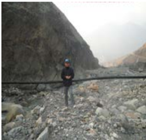
Increased sediments mean relative height of pipe crossing is lower
