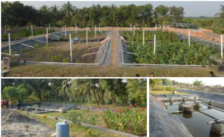
Figure: Vertical flow wetland (top), horizontal flow wetland (bottom left), polishing pond (bottom right)
