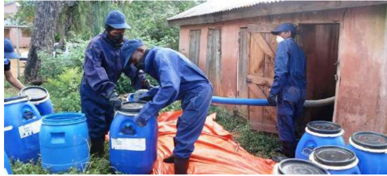
Trained workers use the Gulper to extract sludge from a row of pit latrines at an office building in Ambositra as part of WASHplus's pilot project to test fecal sludge removal tools and business models.
