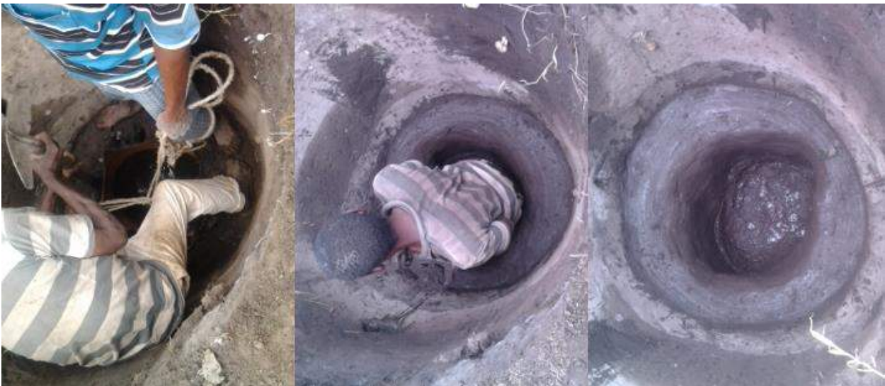
Figure 4: soil cement mixture pit lining
