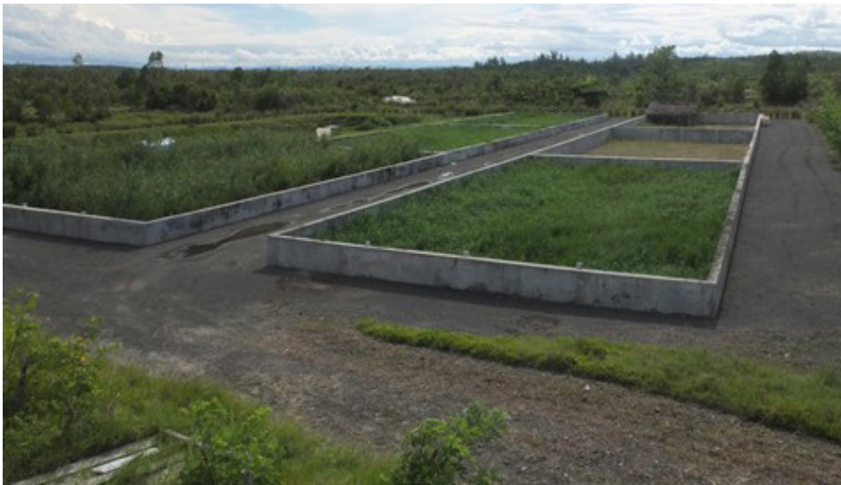
▲ ▼ Treatment plant (humification beds planted with macrophytes) in Toamasina with produced humus.
