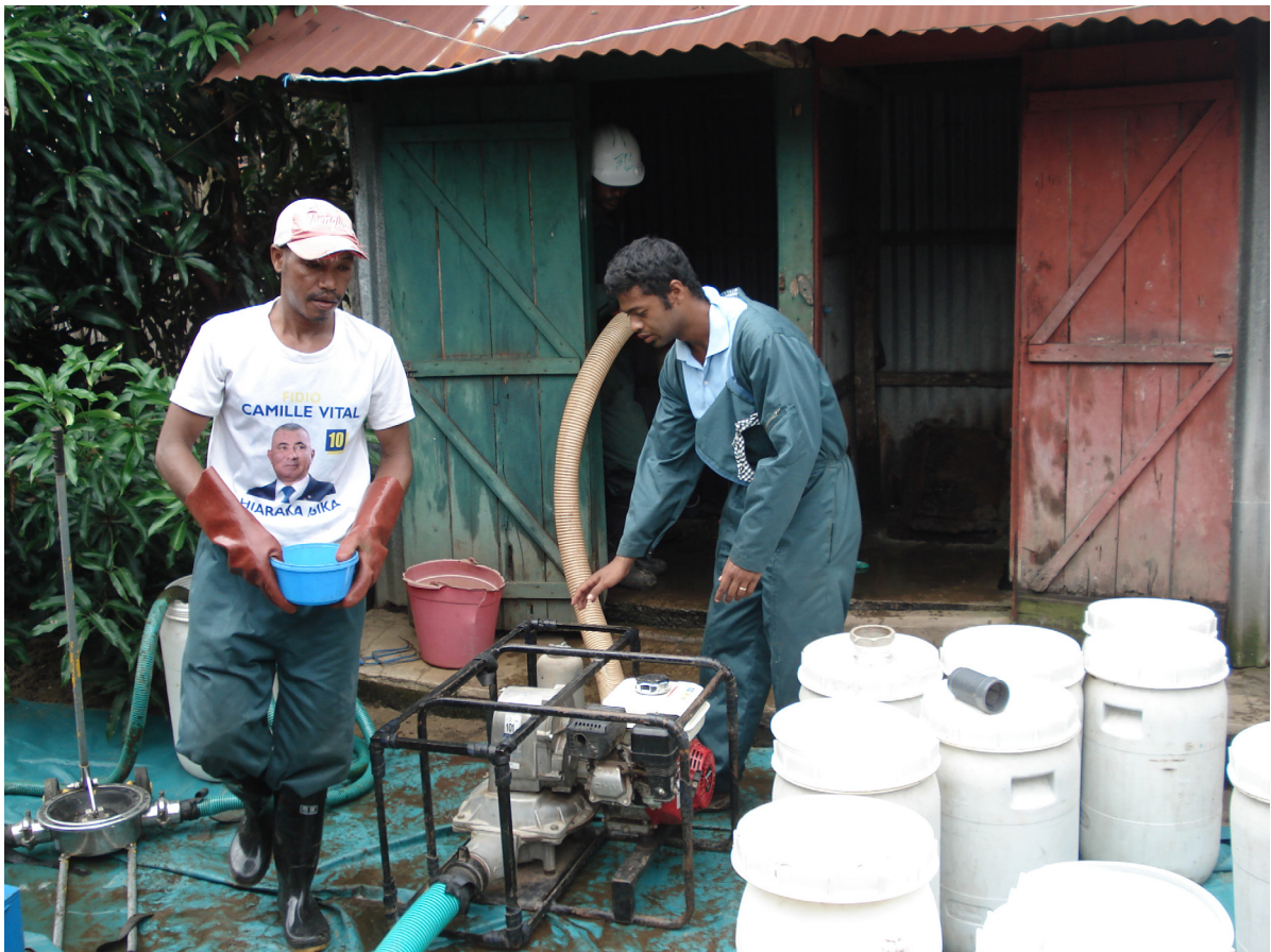
Improved emptying services having access in popular quarters in Toamasina.
