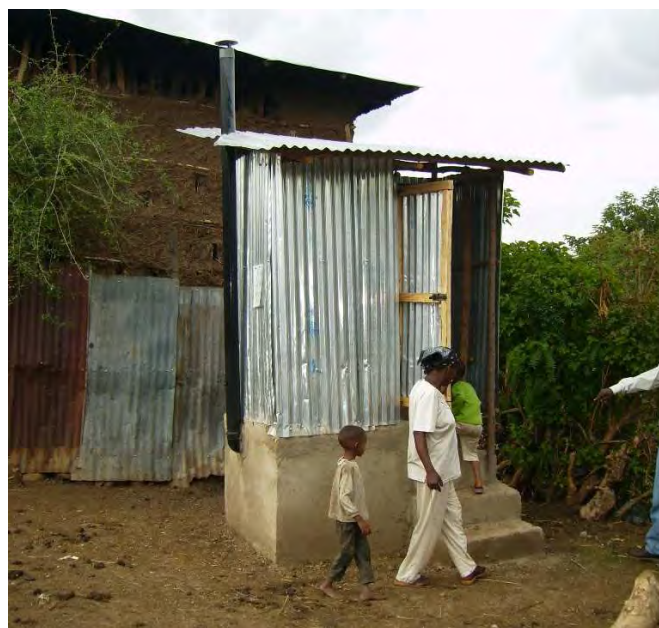
Fig.3: Mr. Agafari's new urine diversion dehydration toilet (source: Wudneh Ayele, 2007)
