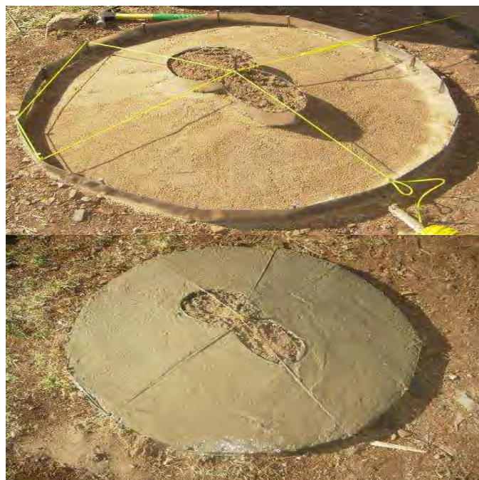
Fig. 7: Arborloo slab construction (source: ROSA Project, 2007)
