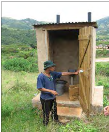
Fig. 4: Double vault UDDT in Maphephetheni in the eThekweni rural area (source: EWS).
