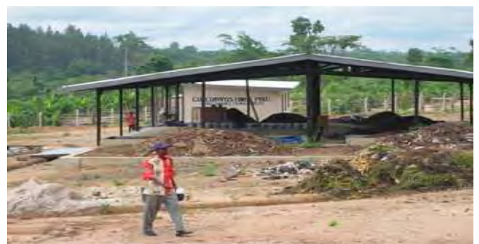
Fig. 3: Co-composting facility (open windrow system) in Kumasi (source: IWMI, 2003).
