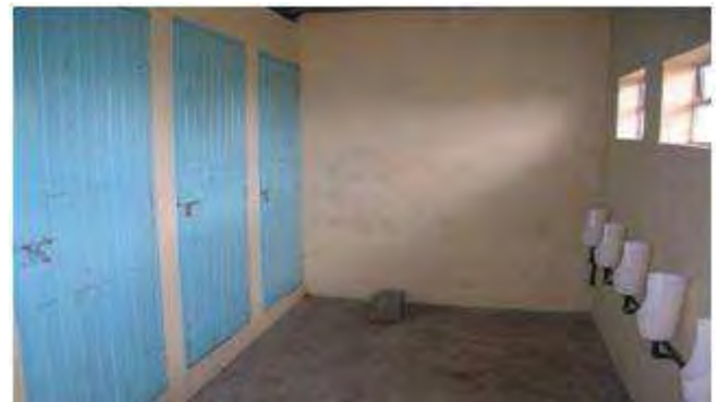
Figure 8 Inside the boys' toilet - 3 cubicles (left) and 6 waterless urinals (right) made of plastic buckets (Source: Muchiri, 2009)
