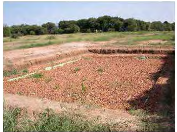
Fig. 7: Constructed wetland (5m x 9m) before greening in 2004 (source: EcoSan Club)
