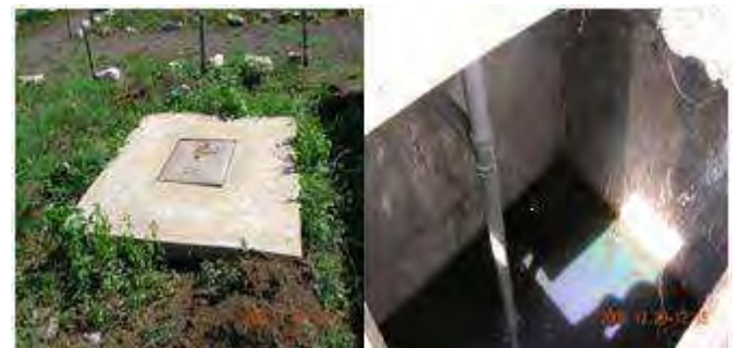
Figure 12 Urine collection tank (2000 L) at Crater View secondary school (Source: Muchiri, 2009)
