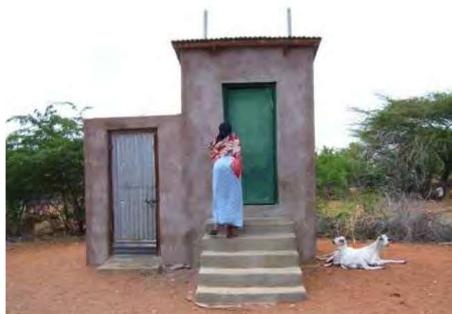
Fig. 5: Household UDDT and shower on the left in the semi-desert area of Wajir, North Eastern Province (source: Paul Mboya, GIZ-Kenya, March 2009).
