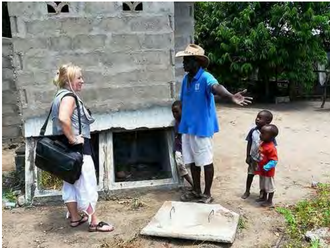
Fig. 11: Discussions about the current state of the UDDTs. This UDDT is no longer in use, note empty faeces vaults and the vault cover on the ground (source: A. Leitner, 2011).
