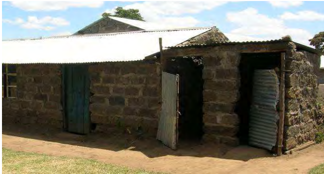
Figure 4 Existing pit latrines
