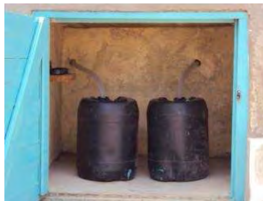
Fig. 8 Urine containers at Mwala Primary School, Ukambani (source: Johannes Orodí, GTZ-Kenya, Oct. 2009)
