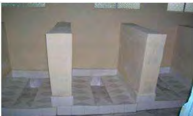
Figure 6 New waterless girls' urinals (squatting) inside the girls' toilet block (Source: Muchiri, 2009)
