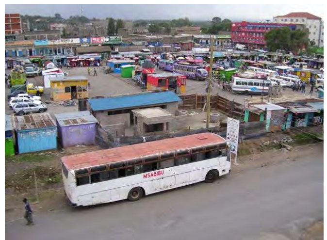
Fig. 3: View of Naivasha bus park with the public toilet at the front of the plot (behind the large bus); during the construction in mid 2007. All photos in this document by C. Rieck (GIZ) in 2008/2009.
