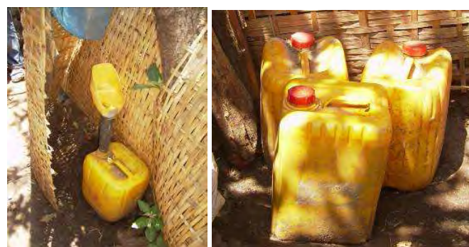
Fig. 9: Waterless urinal (source: ROSA project Arba Minch, 2009).
