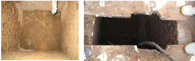
Fig. 6: Both pictures show the single pit family latrine that can be emptied. Left side: this shows the interior of a pit with lined walls. Right side: the pit is shown with opened slab which indicates how the pits can be opened and emptied (source: J. Patinet (2009) Groupe URD).
