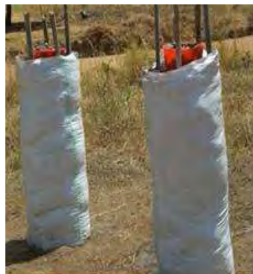
Fig. 3: Two greywater towers in garden in Kitgum (photos by J. Kinobe, 2009).
