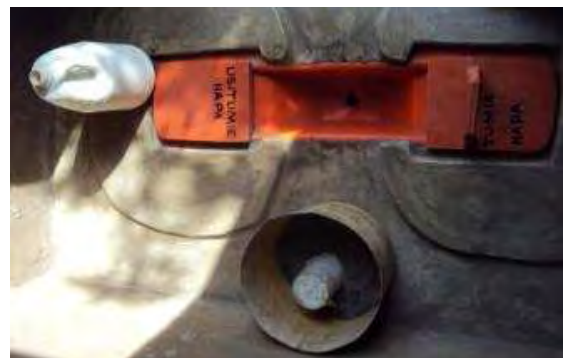
Fig. 6 Plastic UDDT slab for separating urine and faeces inside a UDDT (Source: Laura Kraft, GTZ, June 2010)
