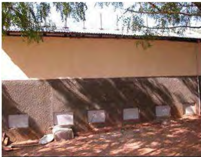
Fig. 6: New "compost" pit latrines for patients, rear view, showing access openings for the removal of faecal sludge (source: EcoSan Club, 2004)
