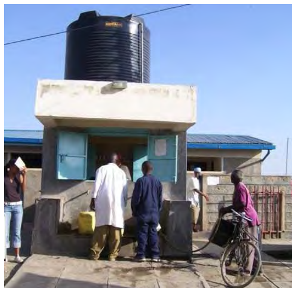
Fig. 5: Customers of the water kiosk. The water tank on the roof holds 5 m 3 (or 250 jerry cans) to bridge water supply gaps for a period of about 1-2 days.
