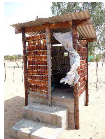
Fig. 5: Ecosan UDD toilet built out of beer cans in Hanahai. The most creative superstructure in the region!
