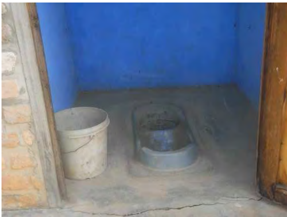
Fig. 9: Inside view of UDDTs at Kiruhura primary school showing plastic urine diversion squatting pan and bucket with ash for covering faeces after defecation. Toilet has been in use for 2.5 years.
