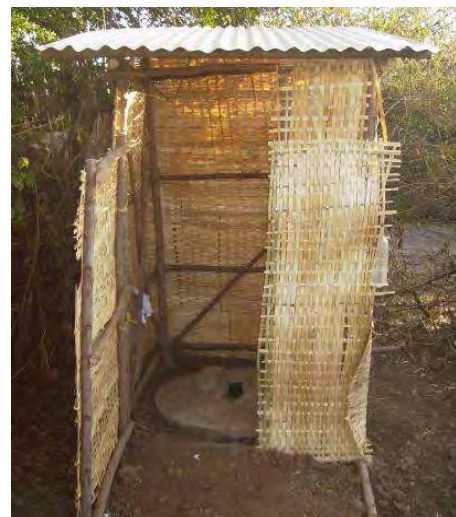
Fig. 3: Typical Arborloo toilet house (source: ROSA Project Arba Minch, 2007)
