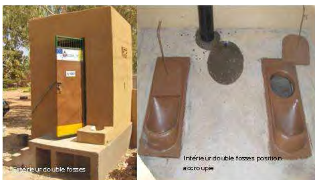
Fig. 7: Outside and inside views of a double vault UDDT with urine diversion squatting pans and anal wash area (dark circle in the middle). Urine jerrycans are stored under the stairs (left picture) (source: CREPA, 2008).
