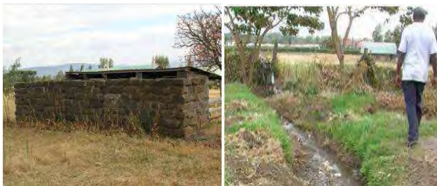
Figure 4 Left: The old pit latrines at Crater view secondary school (Source: Muchiri, 2008) Right: Greywater from kitchen and dish washing was disposed in open drains prior to the project (Source: Raude, 2009)
