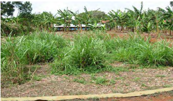
Fig. 11: Constructed wetland, planted with elephant grass (source: EcoSan Club, 2005 – no new photos available but looks more lush now).
