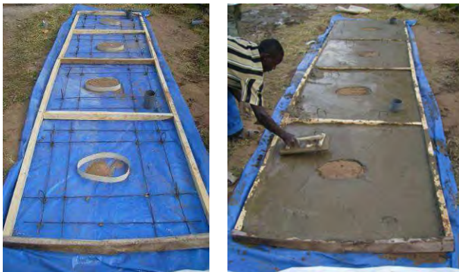
Fig. 5: Fossa alterna slabs during construction (source: ROSA Project, Arba Minch 2007)
