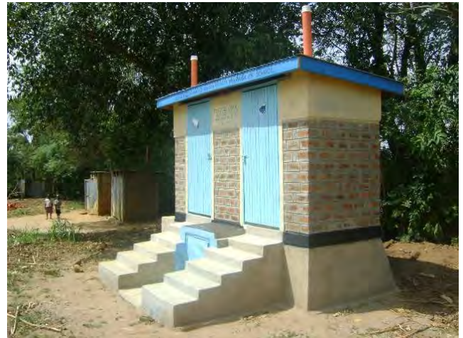
Fig. 5 Newly finished block of 2 school UDDTs. Old pit latrines are visible in the background (Source: Moses Wakala, GTZ, April 2009)
