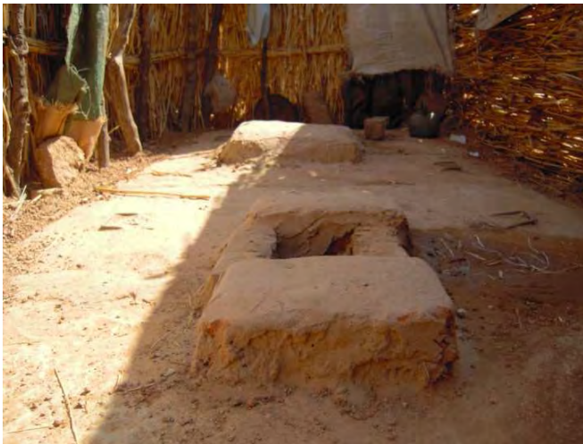
Fig. 7: Double pit family latrine that can be emptied (source: Mahamat Absakine (2010) Groupe URD).
