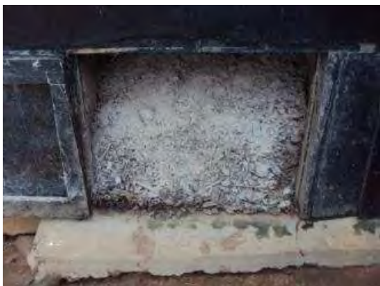
Fig. 7 Faeces vault with ash-covered dried faeces (Source: Laura Kraft, GTZ, June 2010)
