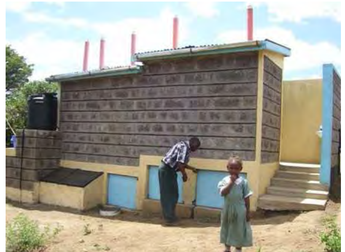
Figure 11 The rear of the UDDT showing the single vaults and the solar drier for the double vault
