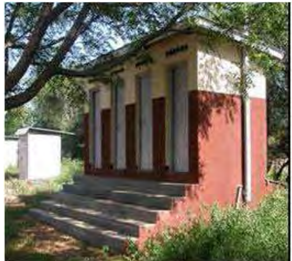
Fig. 4: New UDD toilet block with 4 cubicles for the staff (source: EcoSan Club, 2004)
