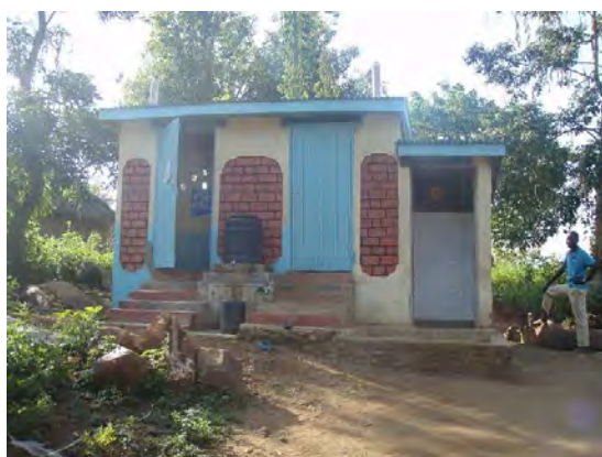
Fig. 16: A double door UDDT with attached shower for a family with more than 20 users in Western Province. The
