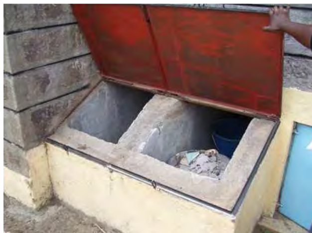
Figure 13 Containers are placed in the solar drier of the double vault compartment (Source: Steffen Blume, 2009)
