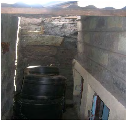
Fig. 9 The rear of the UDDT showing vault doors and a shade for temporary storing the faeces for further drying before utilisation/disposal.
