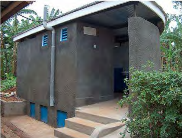
Fig. 6: Demonstration UDD toilet for teachers and visitors, five years old (source: EcoSan Club, 2009)
