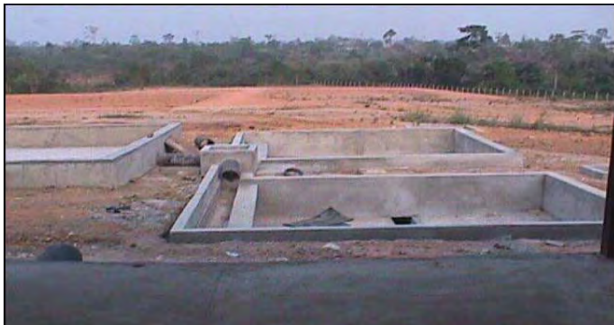
Fig. 4: Faecal sludge drying beds (source: Olufunke Cofie, 2002).
