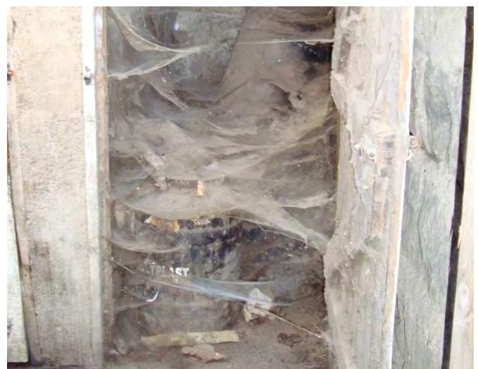
Fig. 12 Old, filled up faeces container stored in the bathroom next to the pit-latrine (Source: L. Kraft, May 2011)
