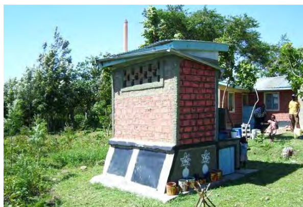
Fig. 6: Back view of household UDDT near Bungoma town in Western Province with two faeces vaults and ventilation pipe (source: Moses Wakala, GIZ-Kenya, Jan. 2010). Note: The inclination of faeces vault doors is not necessary for proper function – see Section 11. Moreover note the toilet is in relative close distance to house.
