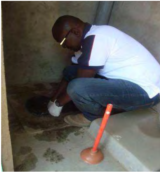
Fig. 8: ROSA project staff unblocking urine pipes at Daraja II primary school UDDT.
