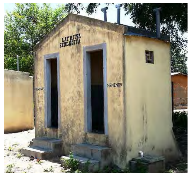
Fig. 7: A public UDDT in Guara-Guara 8 years after construction (source: A. Leitner, 2011).
