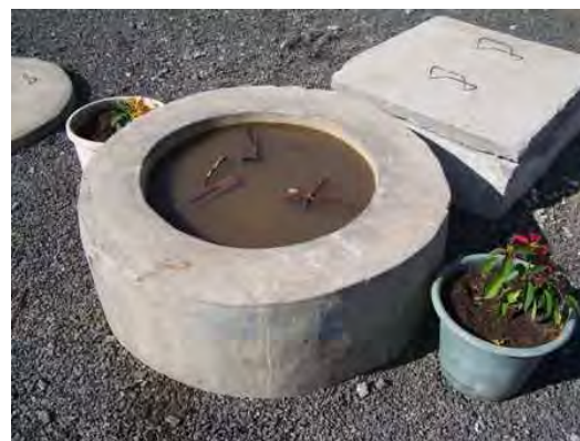
Fig. 8: Area of the top manhole (above biogas fixed dome) of the biogas plant. Clay is used for sealing the lid, and water to keep it wet and thus detect leakages that would show up as bubbles.
