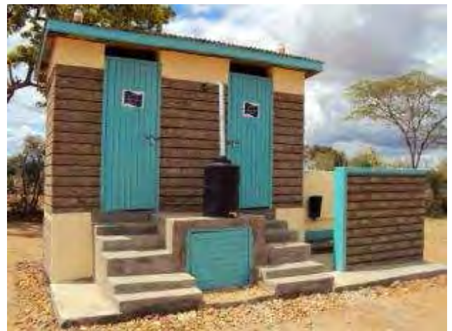
Fig. 3 School UDDTs for boys with urinal at Mwala Primary School near Machakos (source: Johannes Orodí, GTZ-Kenya, Oct. 2009)
