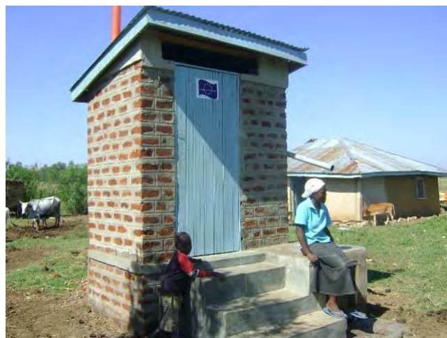
Fig. 3: Rural household UDDT in Nyanza Province (source: Paul Mboya, GIZ-Kenya, Aug. 2009 – Note distance between house and toilet is approx. 20 meters)
