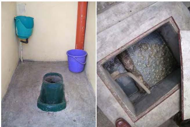
Fig. 6 On the left: Inside the single vault UDDT showing the urine diversion pedestal, men's urinal and a bucket for storing ash. On the right: greywater settling chamber
