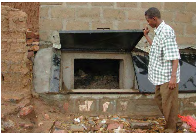
Fig. 5: Faeces vault of UDDT with opening to remove the dried faeces (source: GIZ, 2002).
