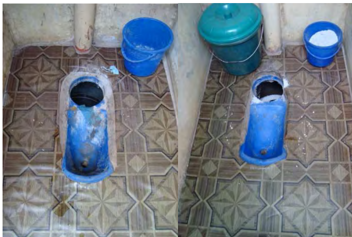
Figure 14 On the left, inside view of toilet used by men with empty ash container, urine on the floor and signs of faecal cross-contamination. Right: Inside view of toilet used by women (Source: L. Kraft, May 2011)
