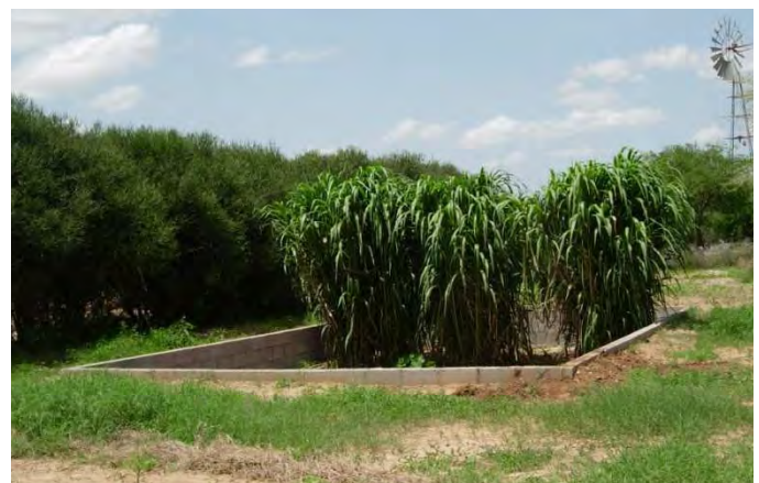
Fig. 8: Constructed wetland in 2006 (source: EcoSan Club)
