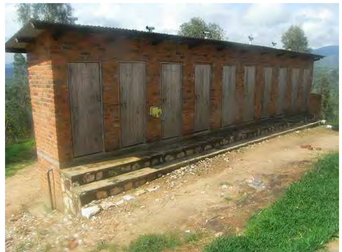
Fig. 6: Toilet block with 10 UDDTs built in Kiziguro primary school (teachers have another 2 UDDTs built separately). Five cubicles are for boys, five for girls.
