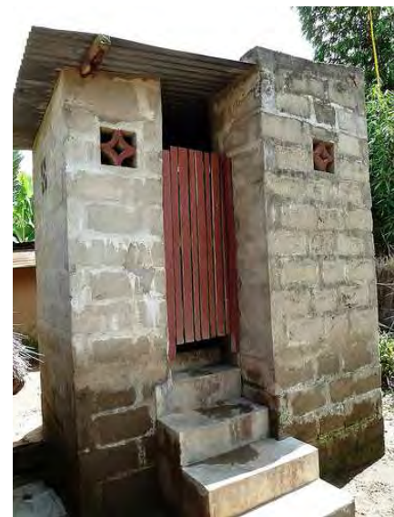
Fig. 3: Well maintained household UDDT in Guara-Guara 8 years after construction (source: A. Leitner, 2011).
