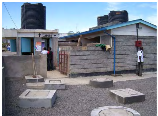
Fig. 3: New public sanitation facility with water kiosk (left side). Underground biogas plant in front.
