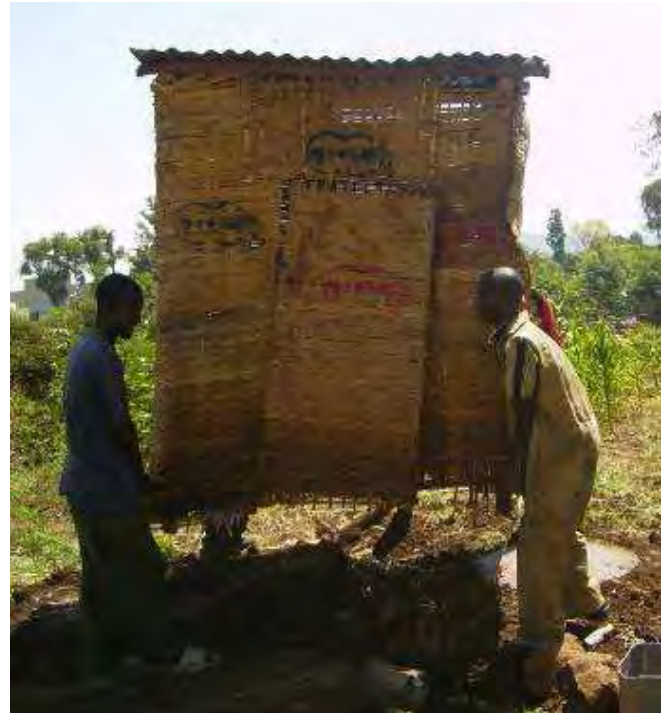
Fig. 4: Portable toilet house (source: ROSA Project Arba Minch, 2008)
