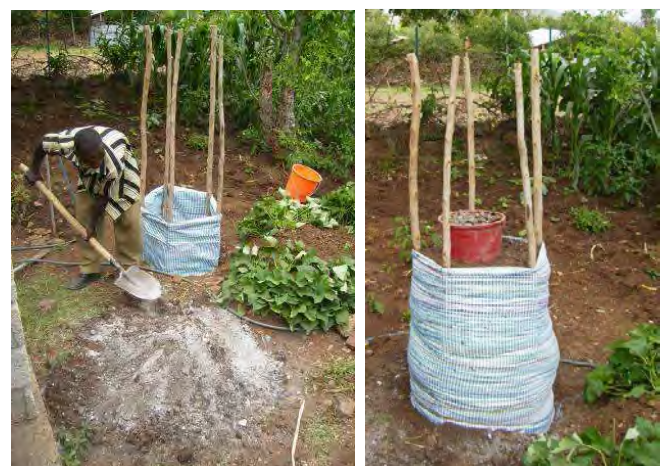
Fig. 6: Left: Mixing soil, compost and ash to fill the tower. Right: Filled greywater tower.
