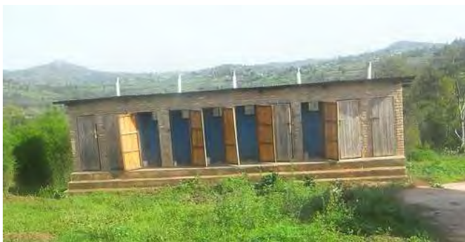
Fig. 5: Toilet block with 10 single vault UDDTs at Kiruhura Primary School (teachers have another 2 UDDTs built separately). Five cubicles are for boys, five for girls 8 .
