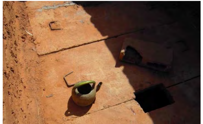
Fig. 8: The slabs of the pit latrines, drop hole is at the bottom right in the shaded part of the photo (source: Mahamat Absakine (2010) Groupe URD). When the document is printed black and white, the drop hole is not visible. Use better photo?
