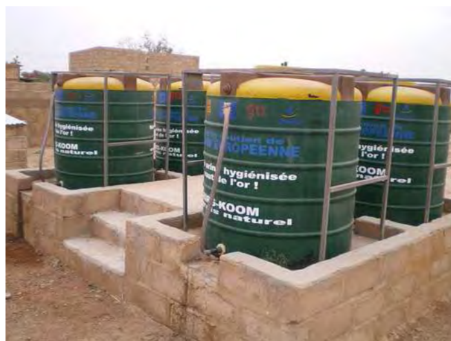
Fig. 8: Eco-station with four 1 m 3 plastic tanks for urine sanitisation (by storage over a period of one month) in sector 27 (source: A. Fall, 2009).
