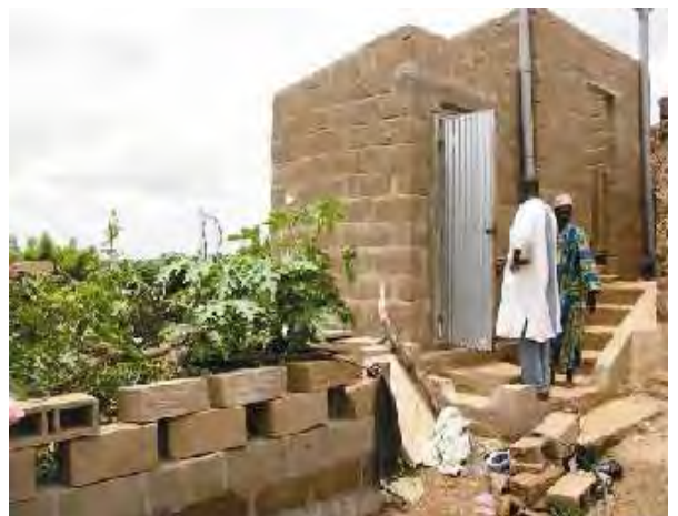
Fig. 3: Ecosan UDD toilet in Koulikoro with shower and greywater garden in 2002 (source: GIZ, 2002).
