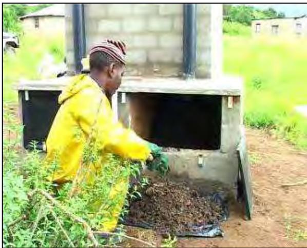
Fig.12: Emptying a UDDT faeces chamber (source: EWS).
