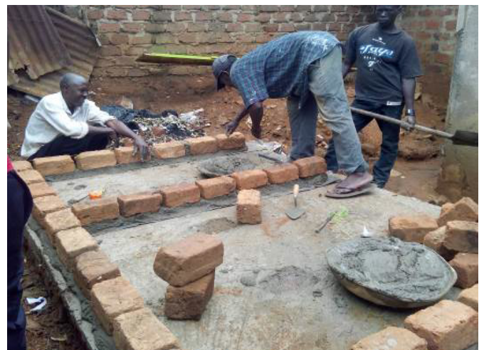
Landlord constructing a lined pit latrine
