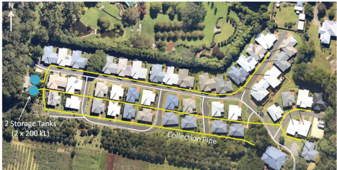
Figure 11.2 Capo di Monte cluster-scale rainwater harvesting system (Courtesy: Bligh Tanner Consulting Engineers, Brisbane, Australia).
