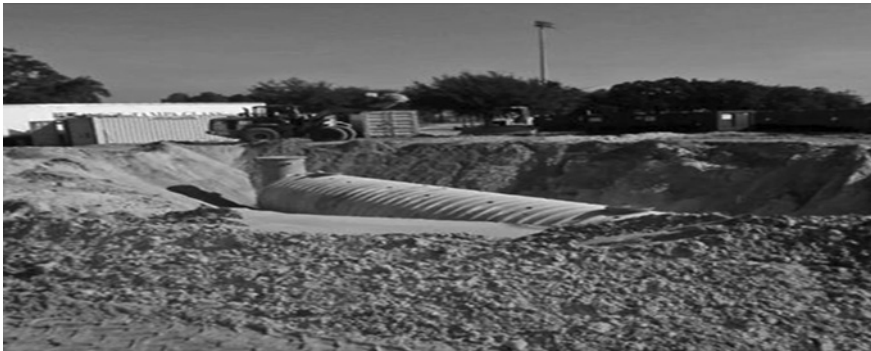
Figure 9.4 Patel Centre cistern installation.
