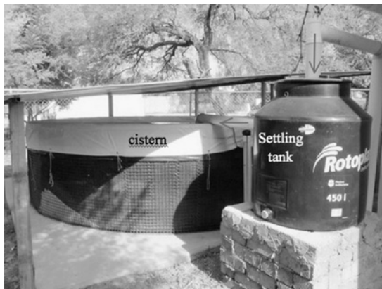
Figure 6.2 Typical above-ground cistern/storage and settling/sedimentation tank.
