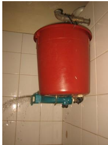
Left: simple solar water heater made from a used 5 litres plastic oil container and painted black on one side. It is placed at a slant to face the sun. The slant also produced a circulation of water within the container. Middle: The shower unit is simply made from a bucket and pipe fittings and can hold about 9 litres of heated water. The water can be heated by the sun, gas or electricity. It makes an excellent shower. Right: the essential candle filter to purify water. This version was made in India, but the candles have been changed several times. The latest candles were made in the UK. The candle filter is an excellent way of purifying water bacteriologically.
