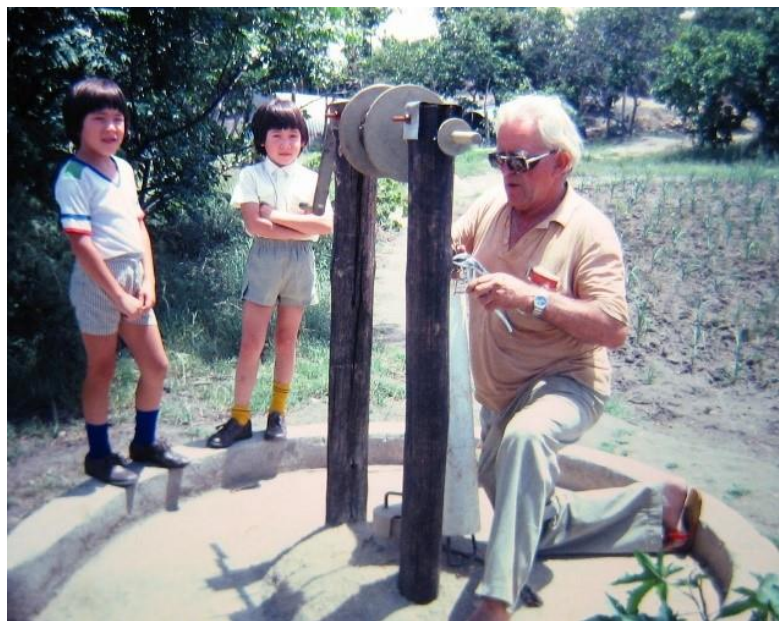
Early hand made bucket pump made of PVC in Epworth work on a tubewell drilled with our own drilling rig. On the right my two young children Paul and Suan admire the Priest Brother Charles, at a mission in Chilimanzi building an early hand built Bucket Pump with a windlass and wooden supports.
