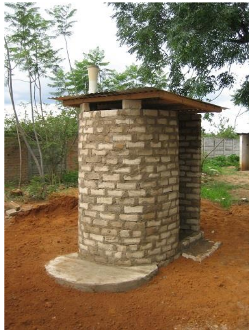
The PVC vent pipe is placed inside the structure of this type of BVIP. The brickwork is built up to the required level and a corrugated iron roof is made with a hole in it for the pipe. Three of these units were built in Epworth during the study. And various methods were used to recycle the contents of the pit. In this case the pit was built from new, but in the other two cases, new slabs were built and mounted on existing full pits, where the pit contents had been removed.
