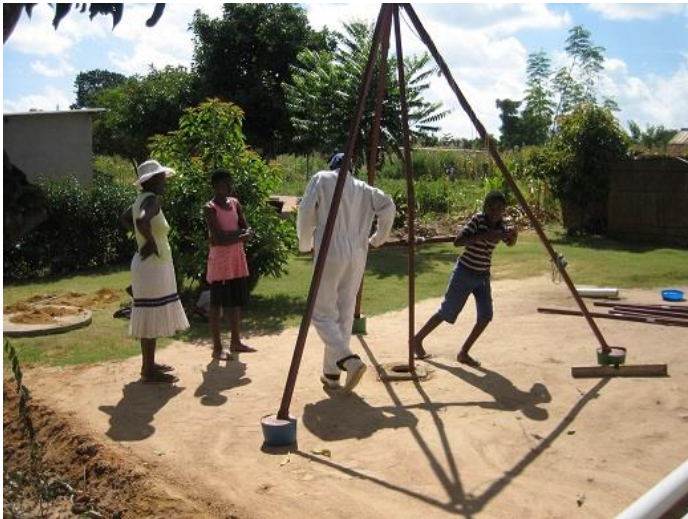
The hole being drilled in Epworth with home-made drilling rig, although the actual auger was made by V&W Engineering.
