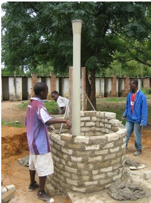
The PVC vent pipe is placed inside the structure of this type of BVIP. The brickwork is built up to the required level and a corrugated iron roof is made with a hole in it for the pipe. Three of these units were built in Epworth during the study. And various methods were used to recycle the contents of the pit. In this case the pit was built from new, but in the other two cases, new slabs were built and mounted on existing full pits, where the pit contents had been removed.
