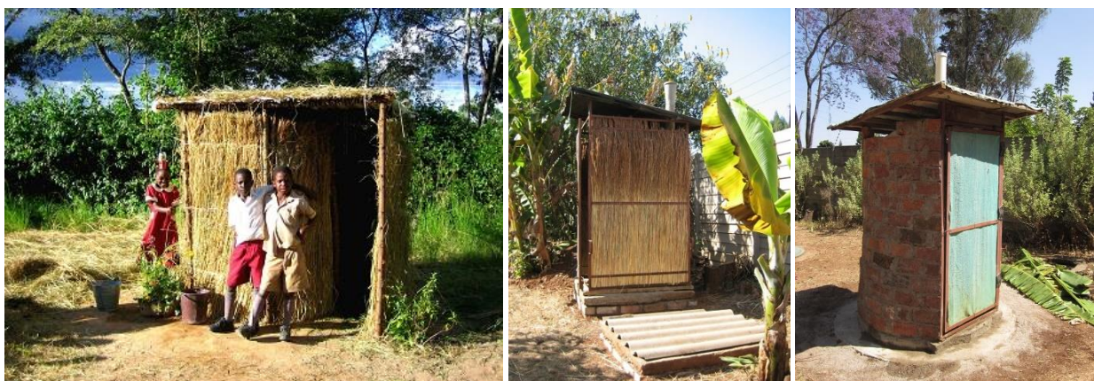
The Arborloo , the Fossa alterna and a hybrid between the Arborloo and the VIP
