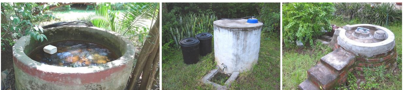
Left: A rainwater harvesting tank for the garden, normally covered by a high density shade cloth. This appears to stop the breeding of mosquitos. Leaves also fall on the shade cloth but the water is just used for gardening. Centre: tank linked to the rain water harvester. Right: tank linked to the kitchen supply.
