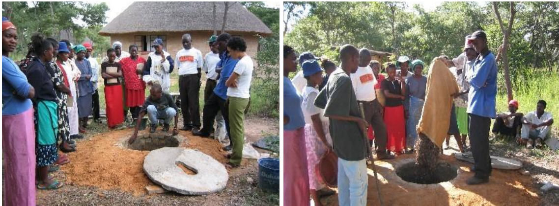
Group of trainees at Kufunda village (Ruwa, Zimbabwe) being taught how to build a simple "compost toilet." Adding leaves to the pit.
