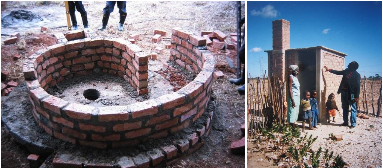
The round and square spiral design built by families with government and donor support during the first two decades after 1980.
