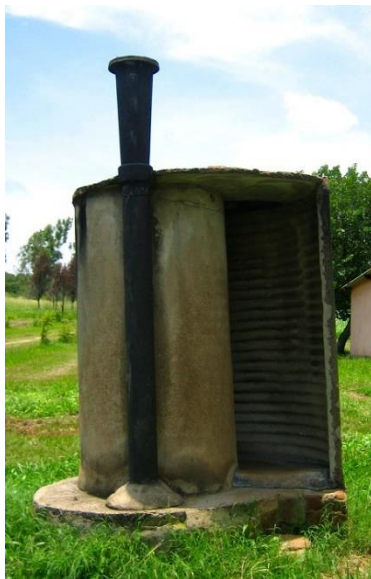
The photo on the left of an early spiral Blair toilet was taken at Henderson in 1976. The photo in the middle was taken of the same toilet in 2010, over 30 years later and still working. The photo on the right was taken in 2010 and still working in 2010. It was also built in 1976. It was fitted with a pedestal.
