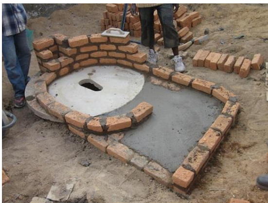
An extension to the slab is made in brick and mortar as shown
