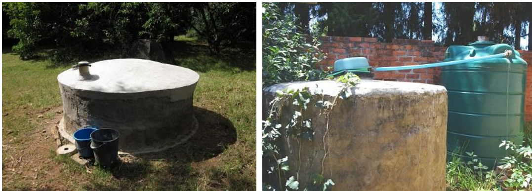
Left: This interesting tank is built from concrete and bricks. Its novel features are the use of shade cloth to reinforce the domed concrete roof and the “bailer bucket” to take water from the tank. Right: a home-made brick tank and a commercially made plastic tank. These rugged plastic tanks are very popular.
