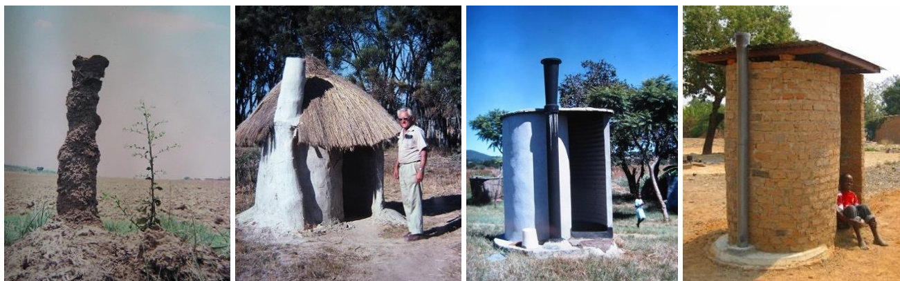
The ant turret – the ultimate ventilator. The ant turret principle is copied in the Blair VIP toilet both old, middle aged and new designs.
