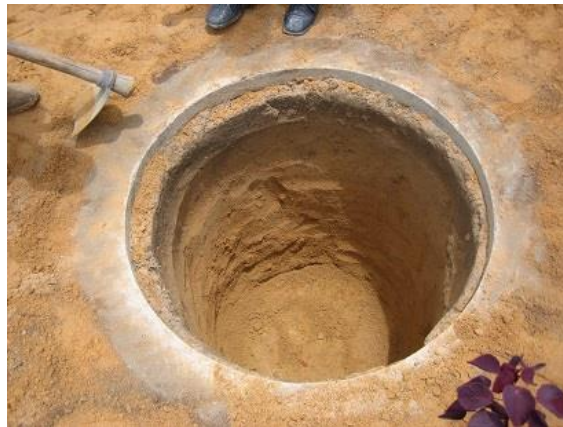
Full hole dug
