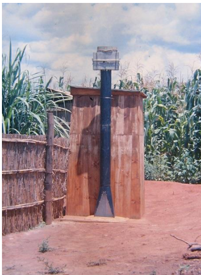
Fly traps were also fitted to the tops of vent pipes. The photos show early experimental Blair toilets built at Henderson Research Station during the early 1970's. Fly behaviour and toilet design were studied in detail during this period.
