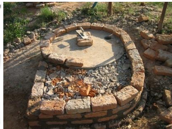
An extension to the slab is made in brick and mortar as shown
