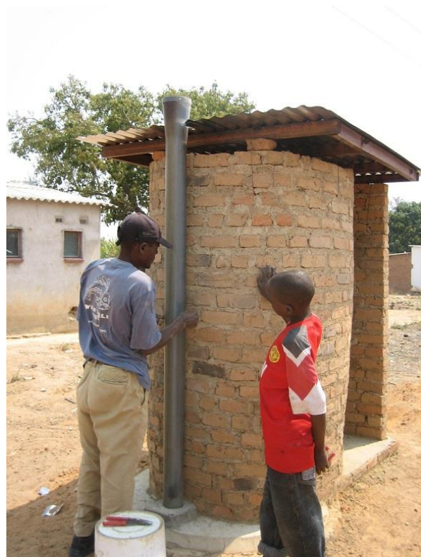
The structure is spiral with a 110mm PVC vent pipe and a roof made of corrugated tin sheet mounted on a treated wooden frame.
