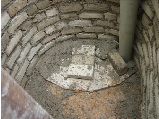
The interior of the toilet. The vent pipe, which is now inside the structure, does not interfere with the use of the toilet. The floor is finally sloped in strong mortar to all wash water to drain into the squat hole. Since the superstructure does not sit on the exposed half of the slab, it can be removed to gain access to the pit.
