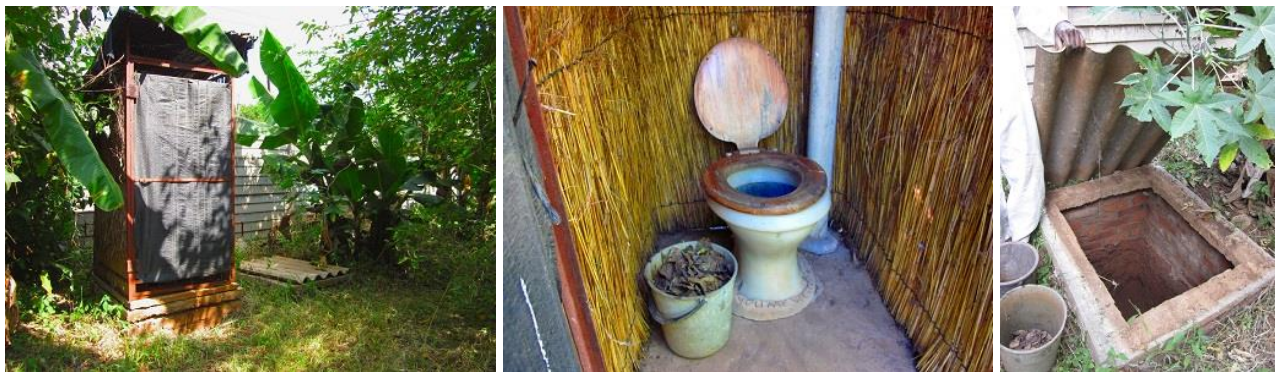
Fossa alterna: This toilet uses two pits alternately. Soil and leaves are added to the pit as well as faeces and urine. The toilet structure, which is portable, is moved from one pit to the other at yearly intervals. When one pit is filling the other is composting.
