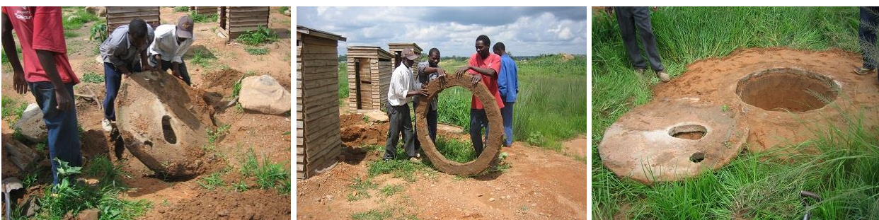
Together with the concrete ring beam it is possible to move all the parts of the Arborloo
