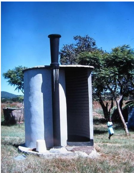
The photo on the left of an early spiral Blair toilet was taken at Henderson in 1976. The photo in the middle was taken of the same toilet in 2010, over 30 years later and still working. The photo on the right was taken in 2010 and still working in 2010. It was also built in 1976. It was fitted with a pedestal.
