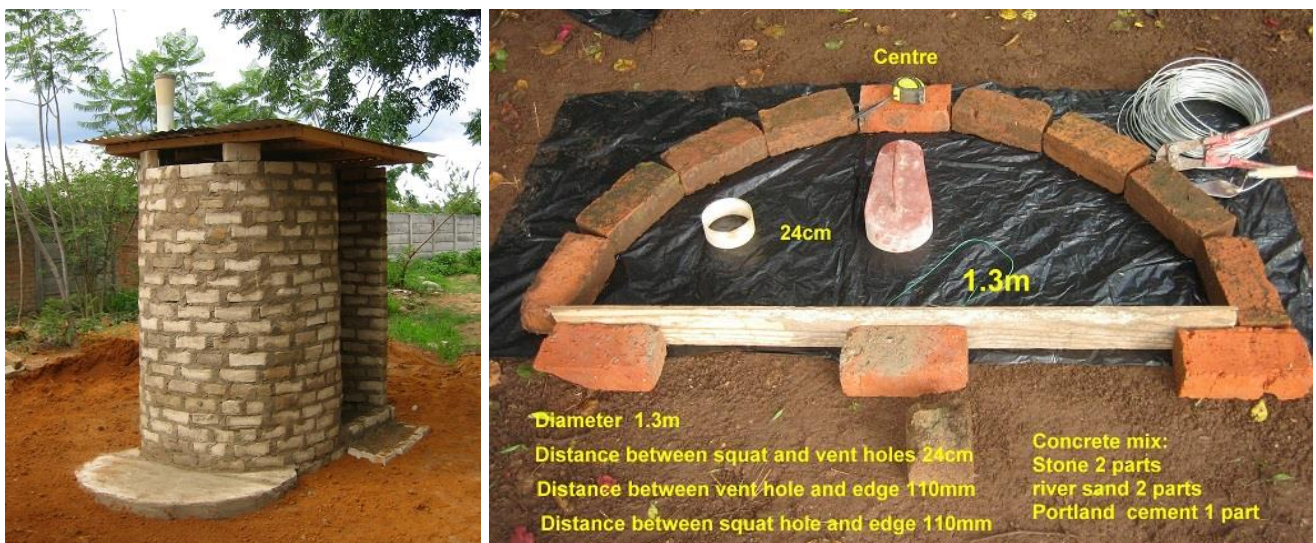
The first prototype of this type of BVIP built at the Chisungu Primary School in Epworth.
