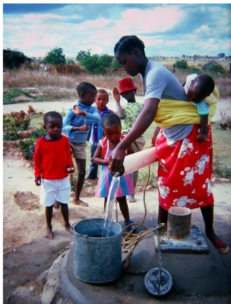
Early hand made bucket pump made of PVC in Epworth work on a tubewell drilled with our own drilling rig. On the right my two young children Paul and Suan admire the Priest Brother Charles, at a mission in Chilimanzi building an early hand built Bucket Pump with a windlass and wooden supports.
