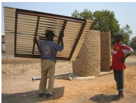
The structure is spiral with a 110mm PVC vent pipe and a roof made of corrugated tin sheet mounted on a treated wooden frame.
