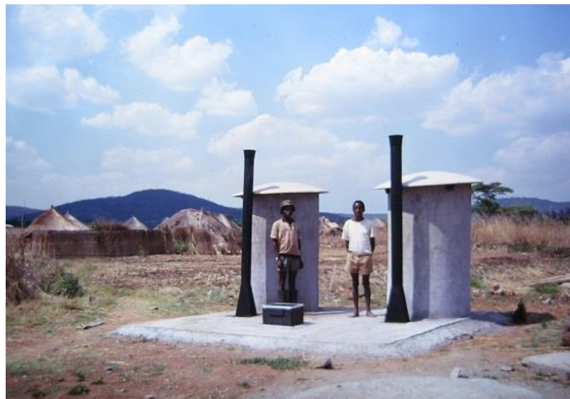
Fly traps were also fitted to the tops of vent pipes. The photos show early experimental Blair toilets built at Henderson Research Station during the early 1970's. Fly behaviour and toilet design were studied in detail during this period.
