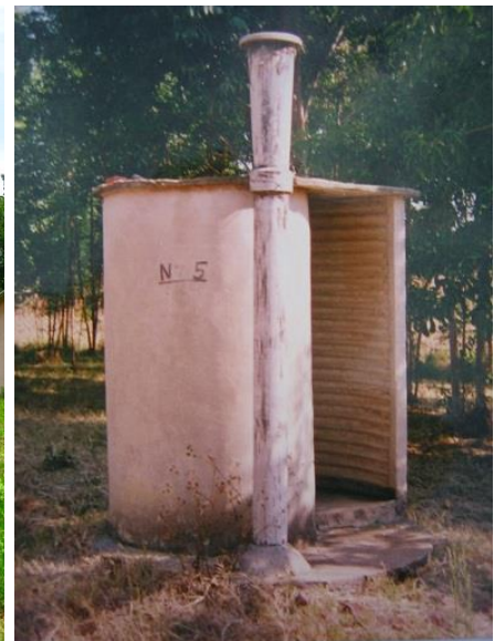
The photo on the left of an early spiral Blair toilet was taken at Henderson in 1976. The photo in the middle was taken of the same toilet in 2010, over 30 years later and still working. The photo on the right was taken in 2010 and still working in 2010. It was also built in 1976. It was fitted with a pedestal.
