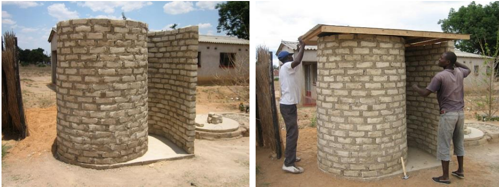
The experimental unit built in Epworth with a fully brick structure on sandy soil
