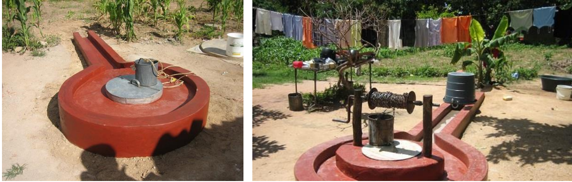
Family well upgraded in the later experimental programme. At first without and then with a windlass.
