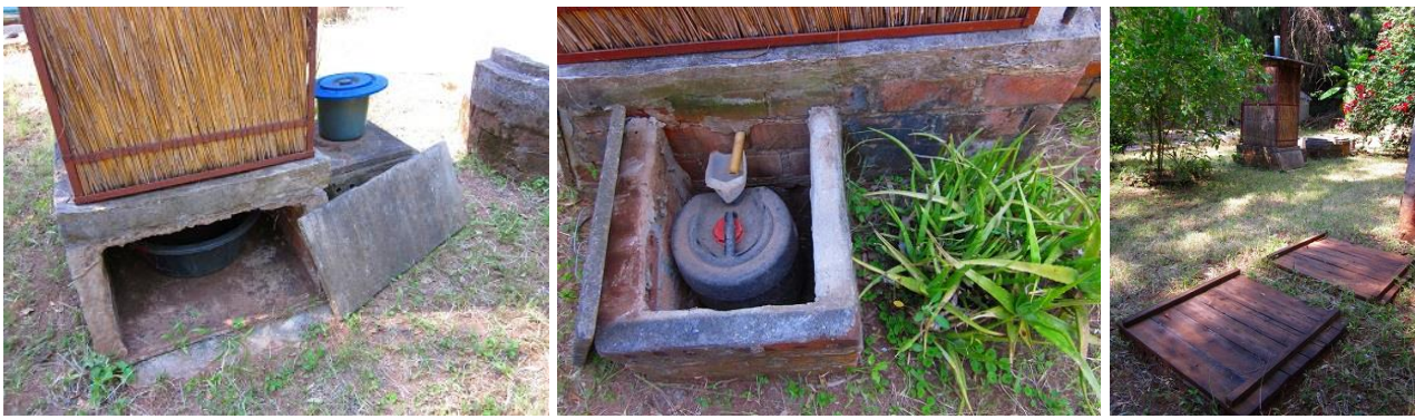
Skyloo: Faecal solids fall into the basin and soil and leaves are added. Urine passes down a pipe into a plastic container. The mix in the basin when nearly full is transferred to a double composting pit (right). Further soil and leaves are added. The mix turns into a good compost. The composting pits are alternated.
