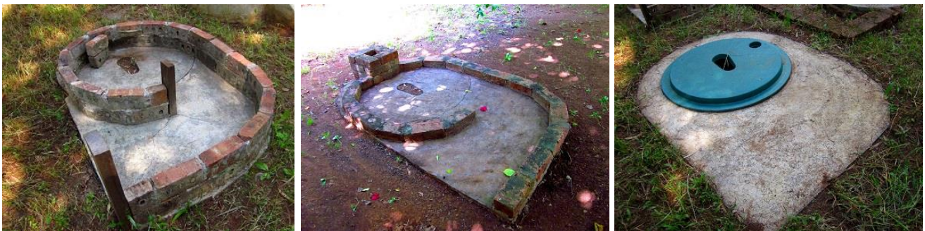
Blair toilet configurations. The spiral structure provides a unit which is stable and semi (but not completely) dark inside. Semi darkness is required for fly control. On the left bricks built on edge. On the right and demonstration of a wide foundation on which the structure is built. An experiment to see if such a broad base will support a brick structure without a pit lining. A pit lining is far preferred.
