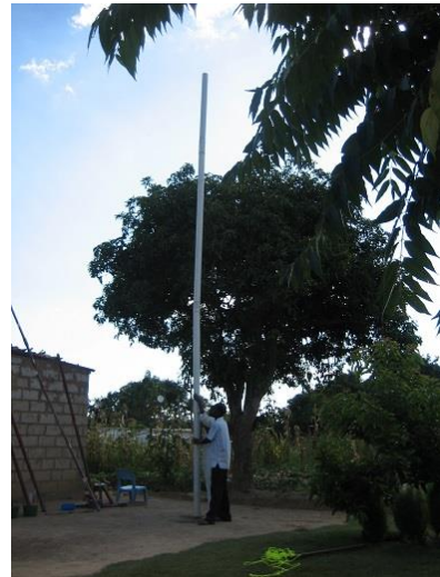
The hole being drilled in Epworth with home-made drilling rig, although the actual auger was made by V&W Engineering.
