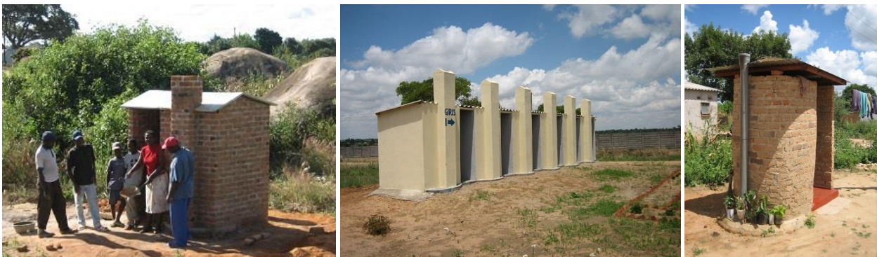
The brick built Blair VIP, the multi-compartment Blair VIP and an upgrade of the uBVIP
