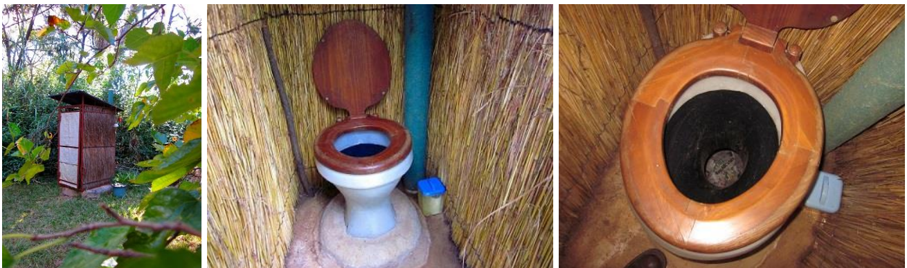
VIP toilet using a door fitted with self-closing hinges. The interior is fitted with a smart pedestal. The unit is completely odourless. Toilet paper kept in container and hand washing facility outside. The structure is made from a steel frame with grass used for walling.
