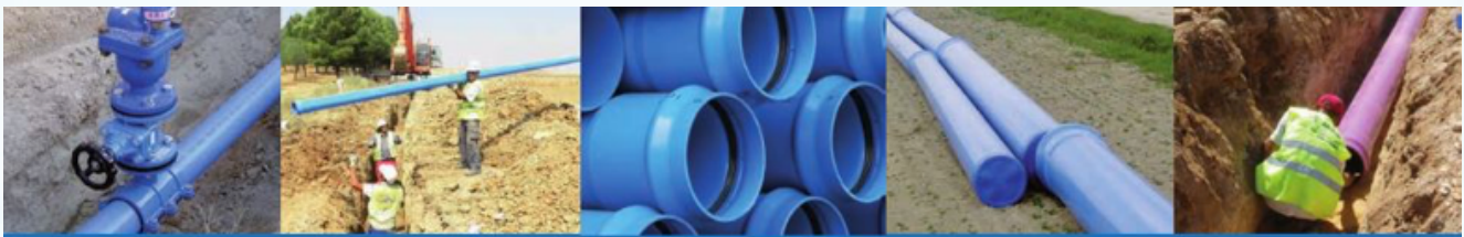
Picture 1: Installation of PCV-BO Pipes
