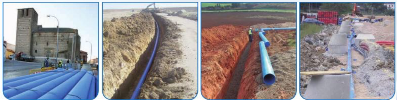
Picture 2: PVC-BO pipes for the transport of drinking water, for the supply of urban and industrial areas, and for filling reservoirs and dams.
