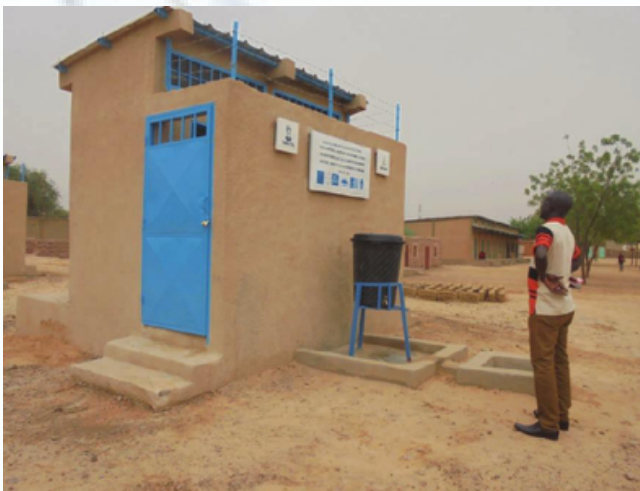
Picture 2: School latrines, a PASEAK deliverable. Picture credit: pS-Eau
