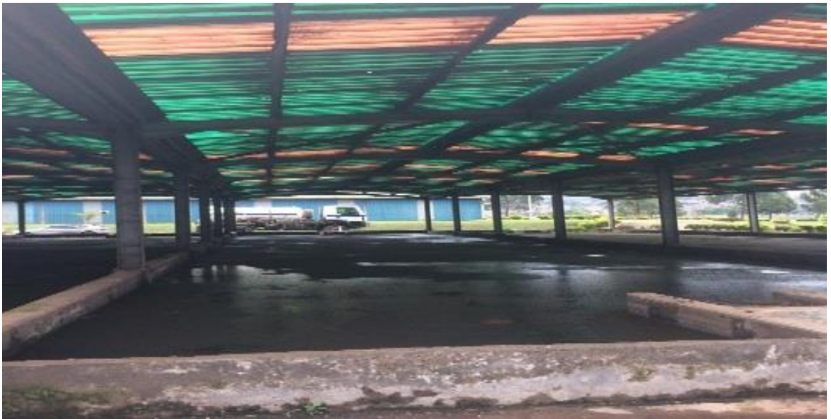
Figure 1: Sludge being dried in one of the unplanted covered sludge drying beds at LSTP, Kampala, Uganda.
