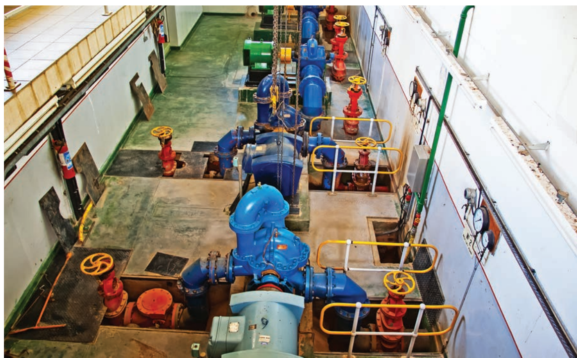
The low electricity generation capacity in many African towns and cities negatively affects wastewater treatment
