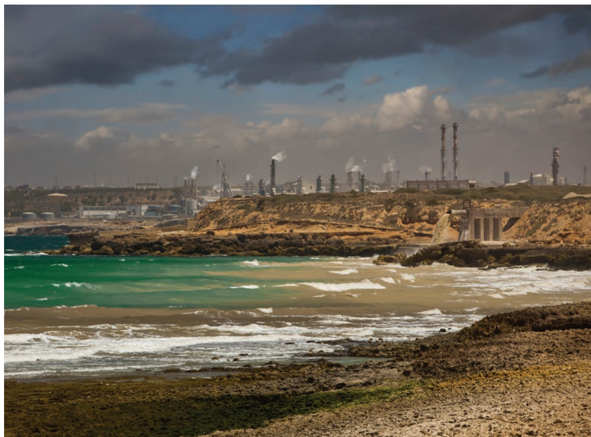
Poor water and wastewater infrastructure, inadequate solid waste management and poorly managed faecal sludge management lead to land and water contamination
