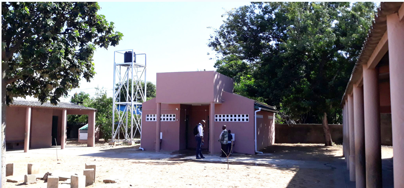
Image 3: School washblock in Maputo, Mozambique Credit: WSUP
