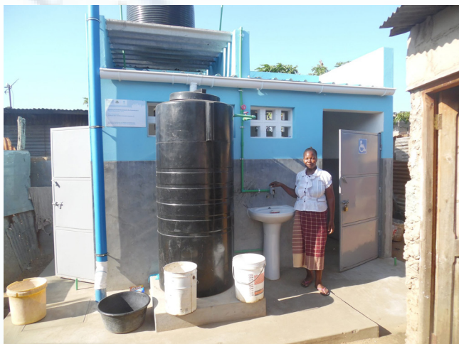
Image 2: Resident uses a communal washblock in Maputo, Mozambique. Credit: WSUP
