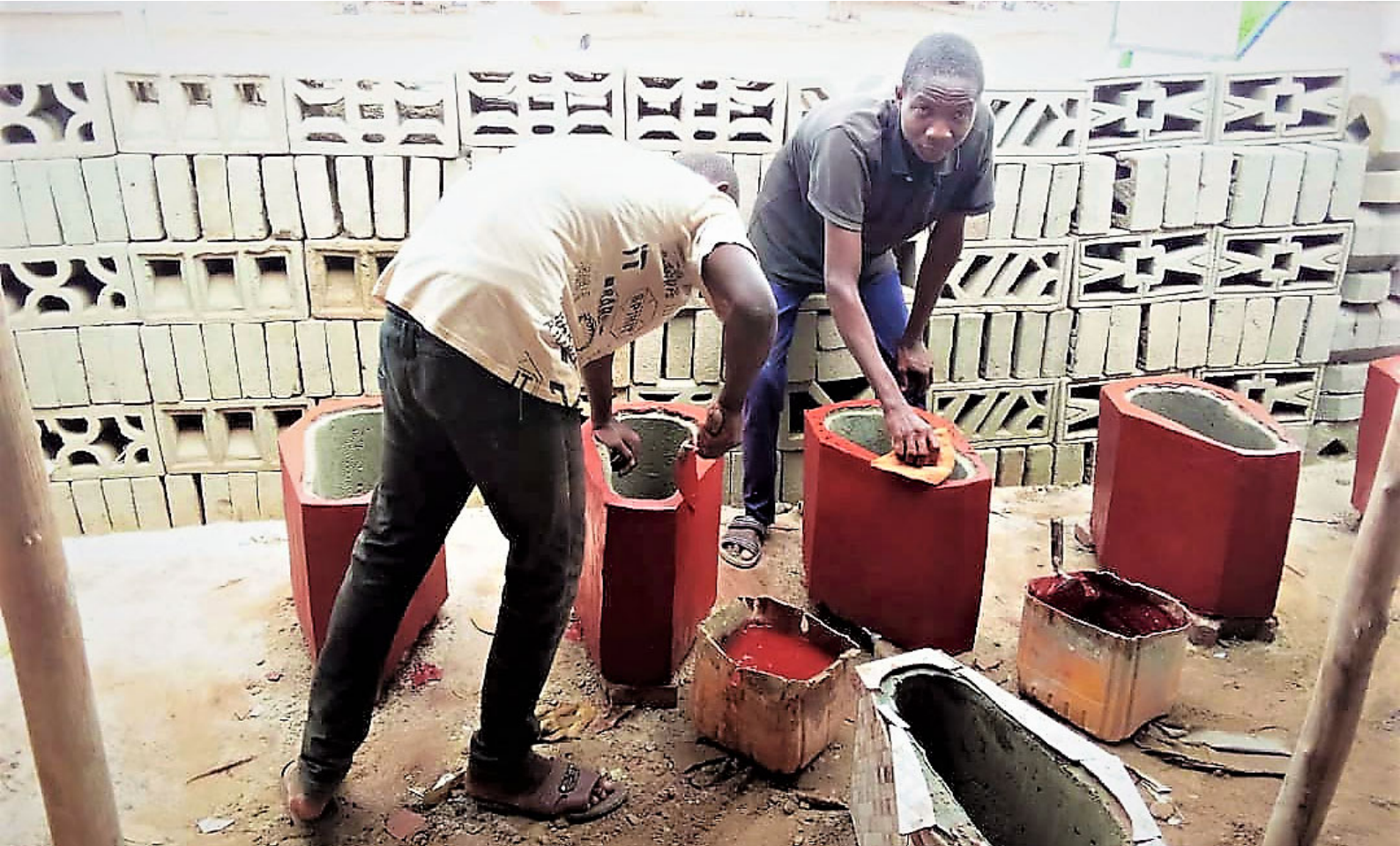
A mason building seated toilets © MuniWASH Benin
