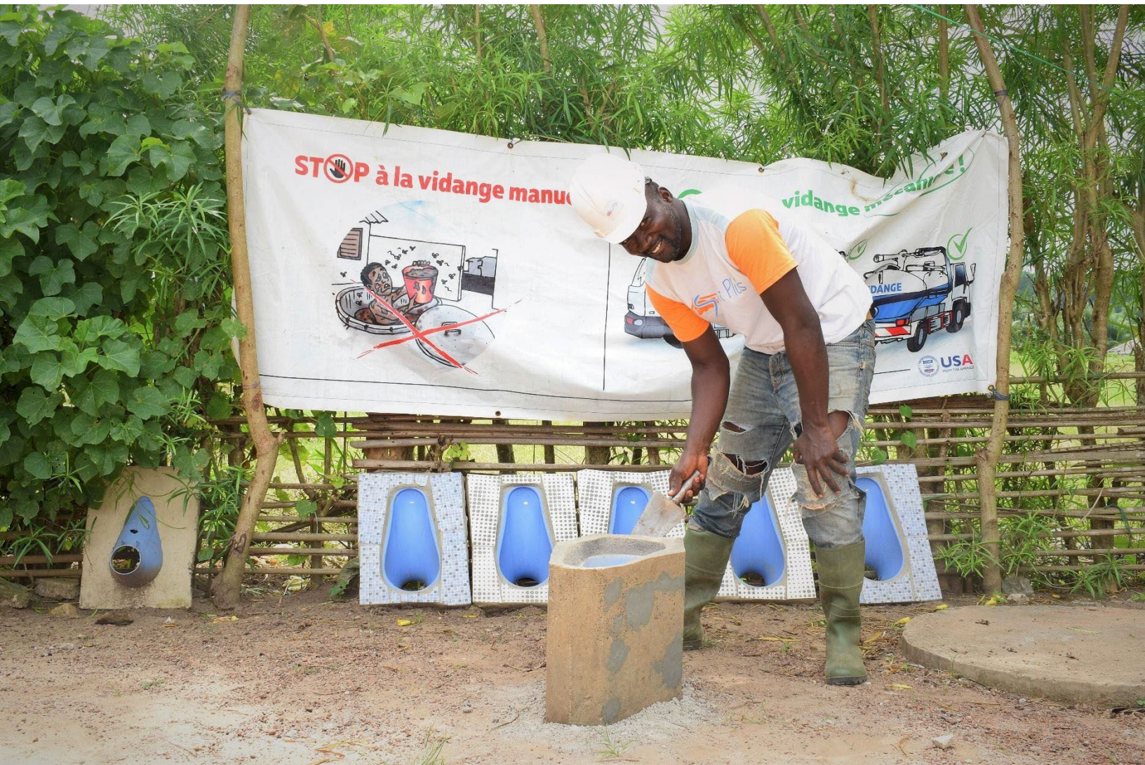
A MICRO SANITATION CONTRACTOR BUILDS A PREFABRICATED LATRINE © MUNIWASH/ - CÔTE D'IVOIRE
