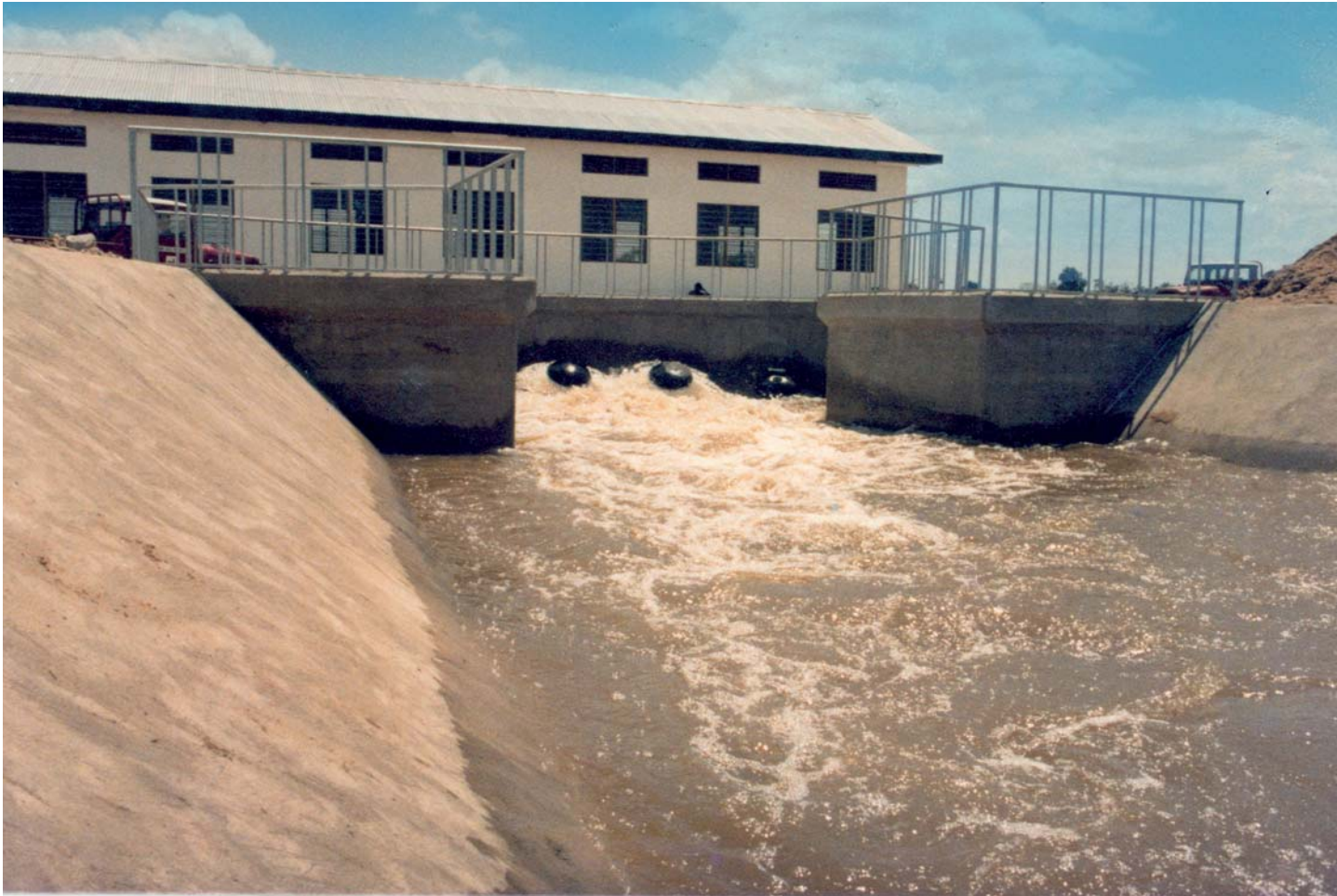
Dam near Shinyanga, Northern Tanzania
