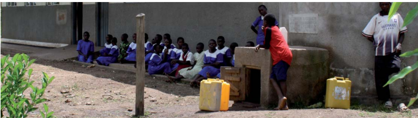
Rainwater Harvesting at a school in Uganda
