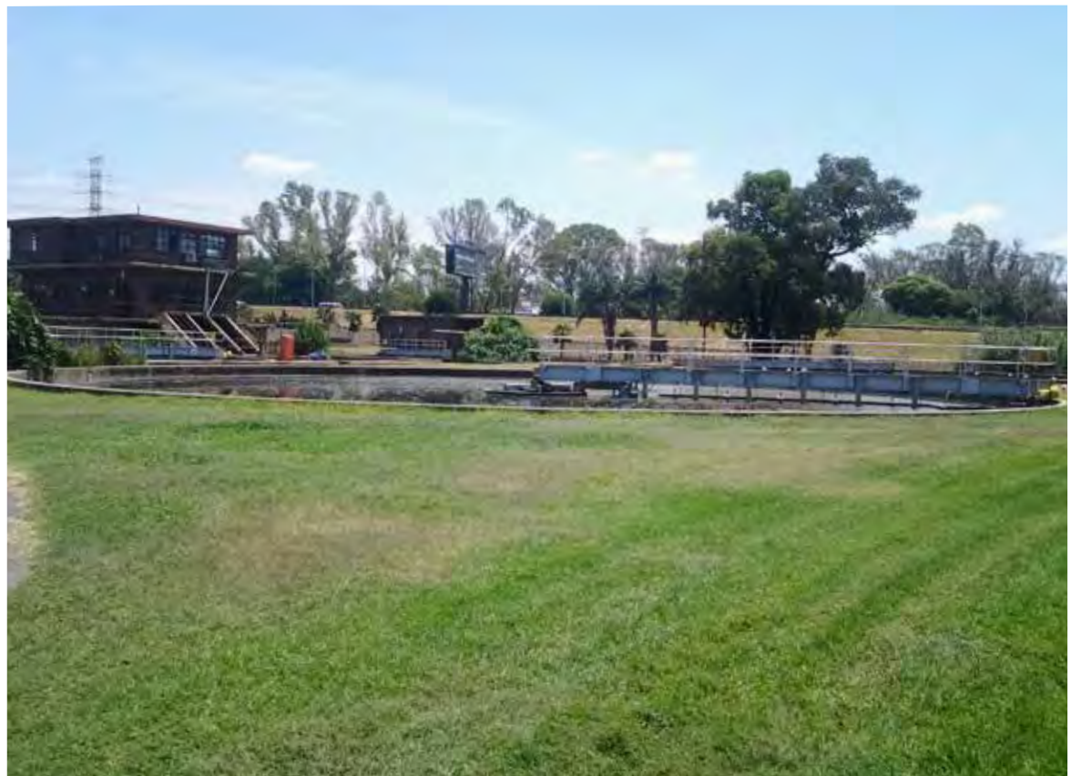
Reuse of wastewater to water lawns
