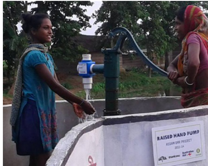
Figure 8. PurAll Handpump chlorinator (Source: EaSol Private Limited)
