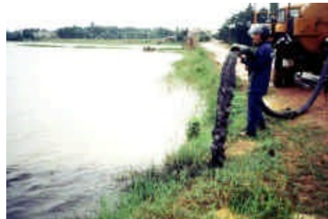
Photo 2 Discharge of untreated septage into a fishpond in Vietnam
