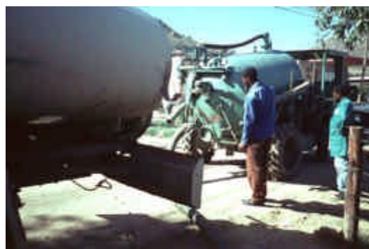
Photo 4 Transboarding of FS from a Mini-Tanker to A Standard-Size Vacuum Tanker (Maseru, Lesotho)
