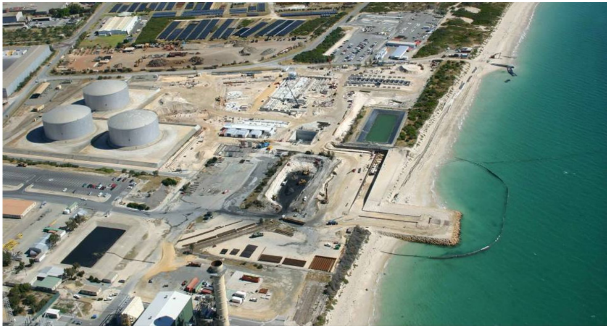
Figure 3: Aerial photo of the Perth Seawater Desalination Plant in Perth, Western Australia. This plant uses reverse osmosis to desalinate seawater.
