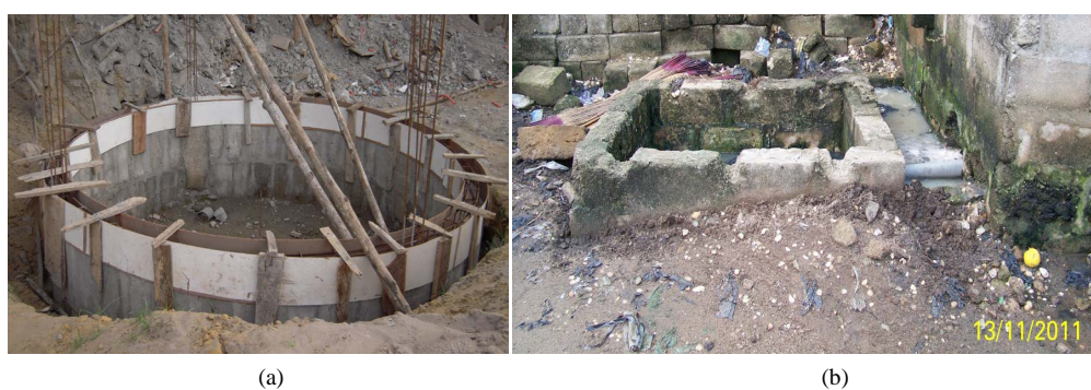
Figure 6. Soakaway pit. (a) under construction (b) current never emptied.
