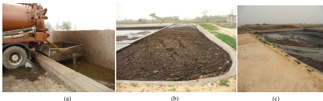
Figure 9. The treatment plant. (a) The grit chamber; (b) The anaerobic pond; (c) From the third WSP to the sea.
