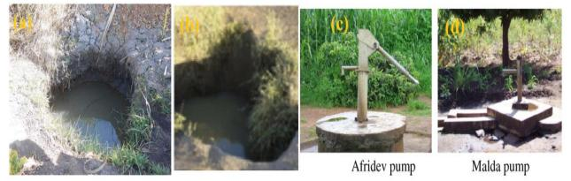
**Figure 2** Surface water source (a), unprotected shallow well (b), borehole (c) and (d). Source (Pritchard, Mkandawire et al. 2008, Mkwate, Chidya et al. 2017, Smiley 2017)
